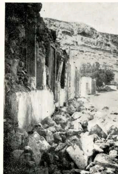
Fig. 1. — Common earthquake failures in the southern part of the Central Crete during the Earthquake of May 14, 1959. Above, wall cracks to houses with flat heavy earthen roofs built upon thin alluvium in Pitsidia. Below, ruins of houses resting on alluvium 80-100 m from the sea-shore of Matala. See in the background of the left picture houses built on limestones left intact. (Photos by M. Karatarakis)
