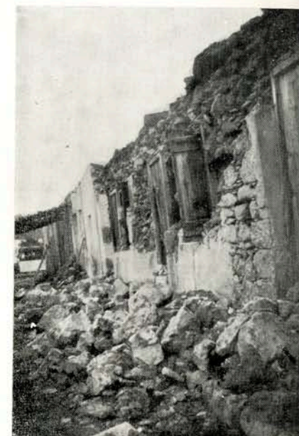
Fig. 1. — Common earthquake failures in the southern part of the Central Crete during the Earthquake of May 14, 1959. Above, wall cracks to houses with flat heavy earthen roofs built upon thin alluvium in Pitsidia. Below, ruins of houses resting on alluvium 80-100 m from the sea-shore of Matala. See in the background of the left picture houses built on limestones left intact. (Photos by M. Karatarakis)
