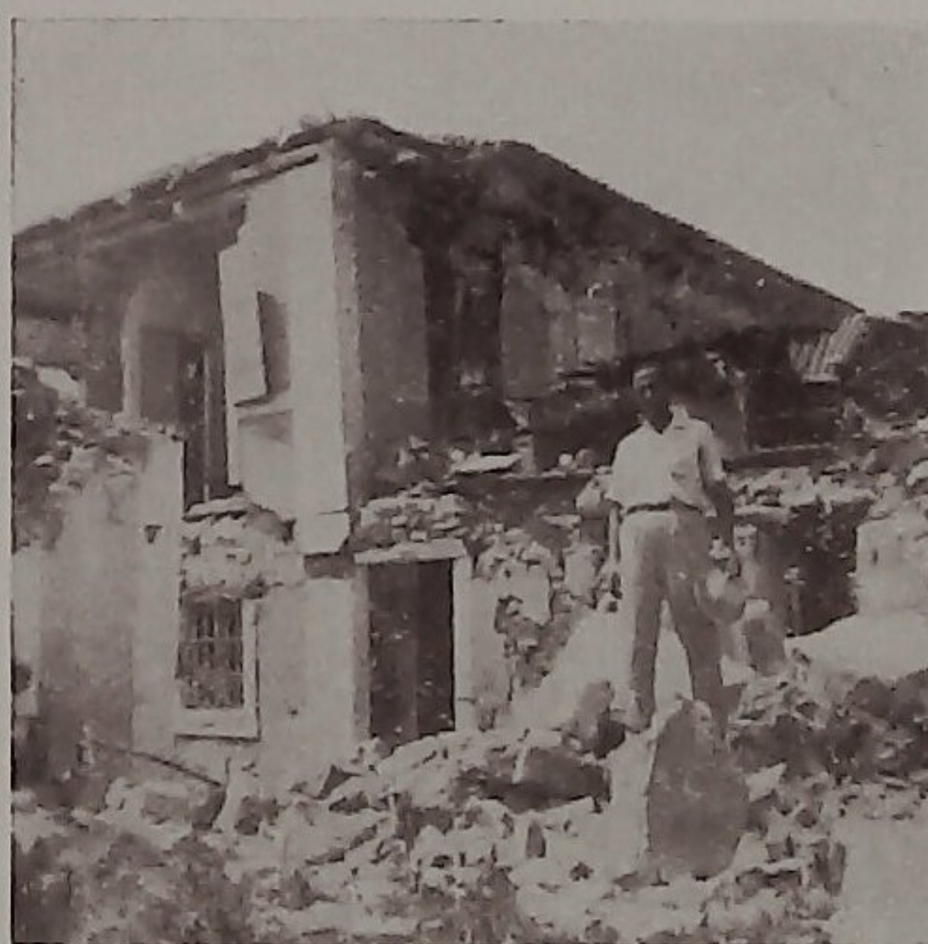
Fig. 11.—Common type of earthquake failure in Lixuri ascribed largely to the poor construction.
