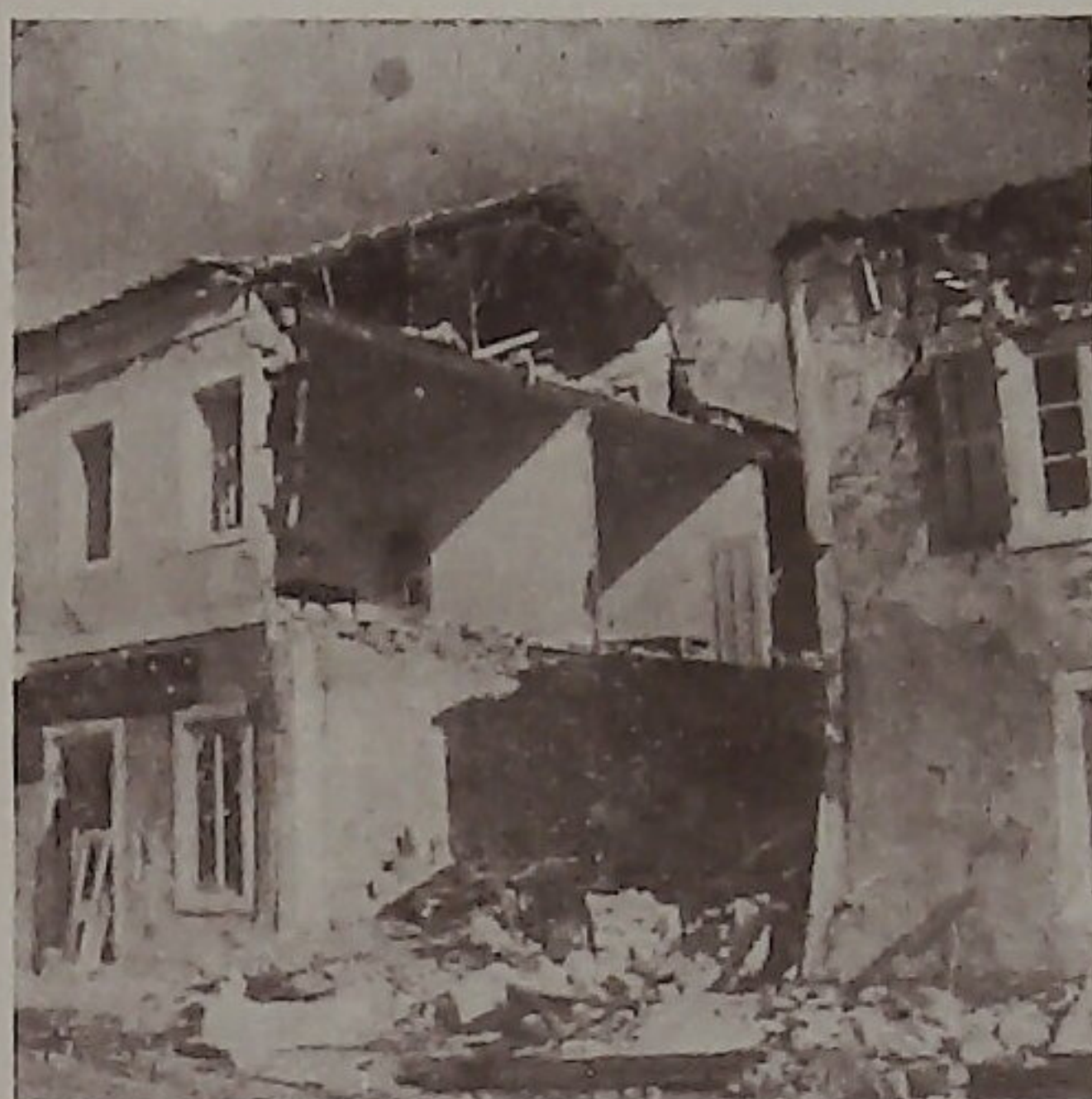
Fig. 5.—«Petrifaction» of a wall motion during the earthquake in Vathy (Ithaca).
