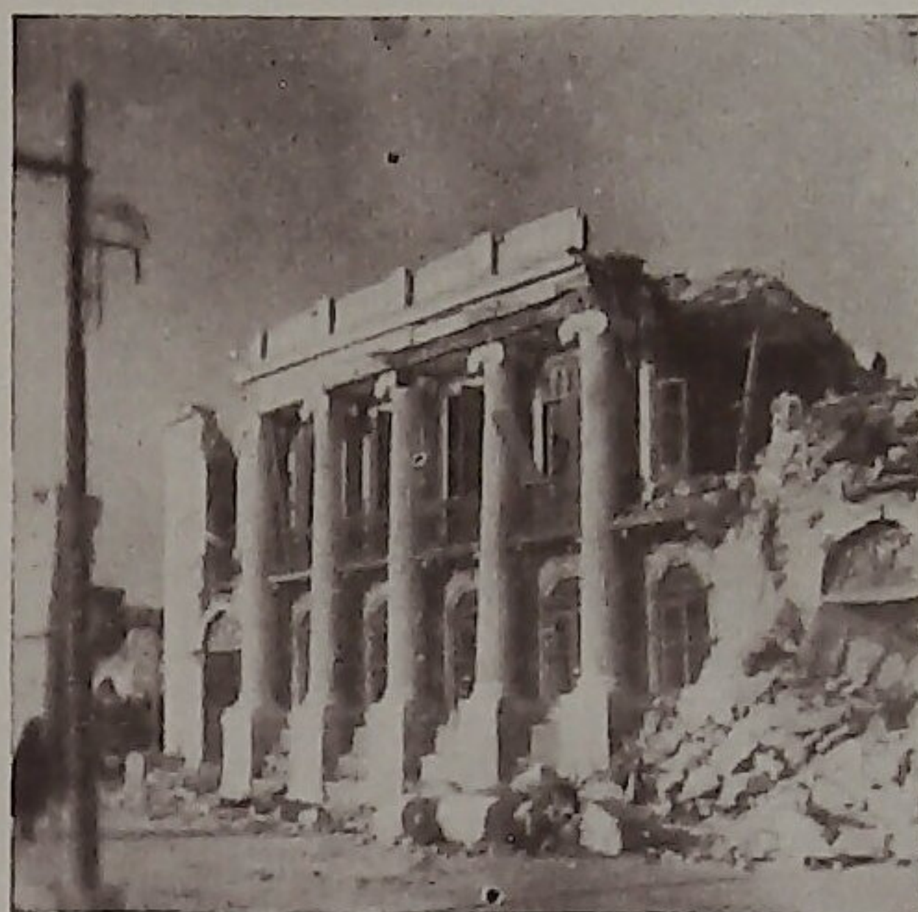
Fig. 9.—Severe damage to the Ionian Bank in Argostoli.
