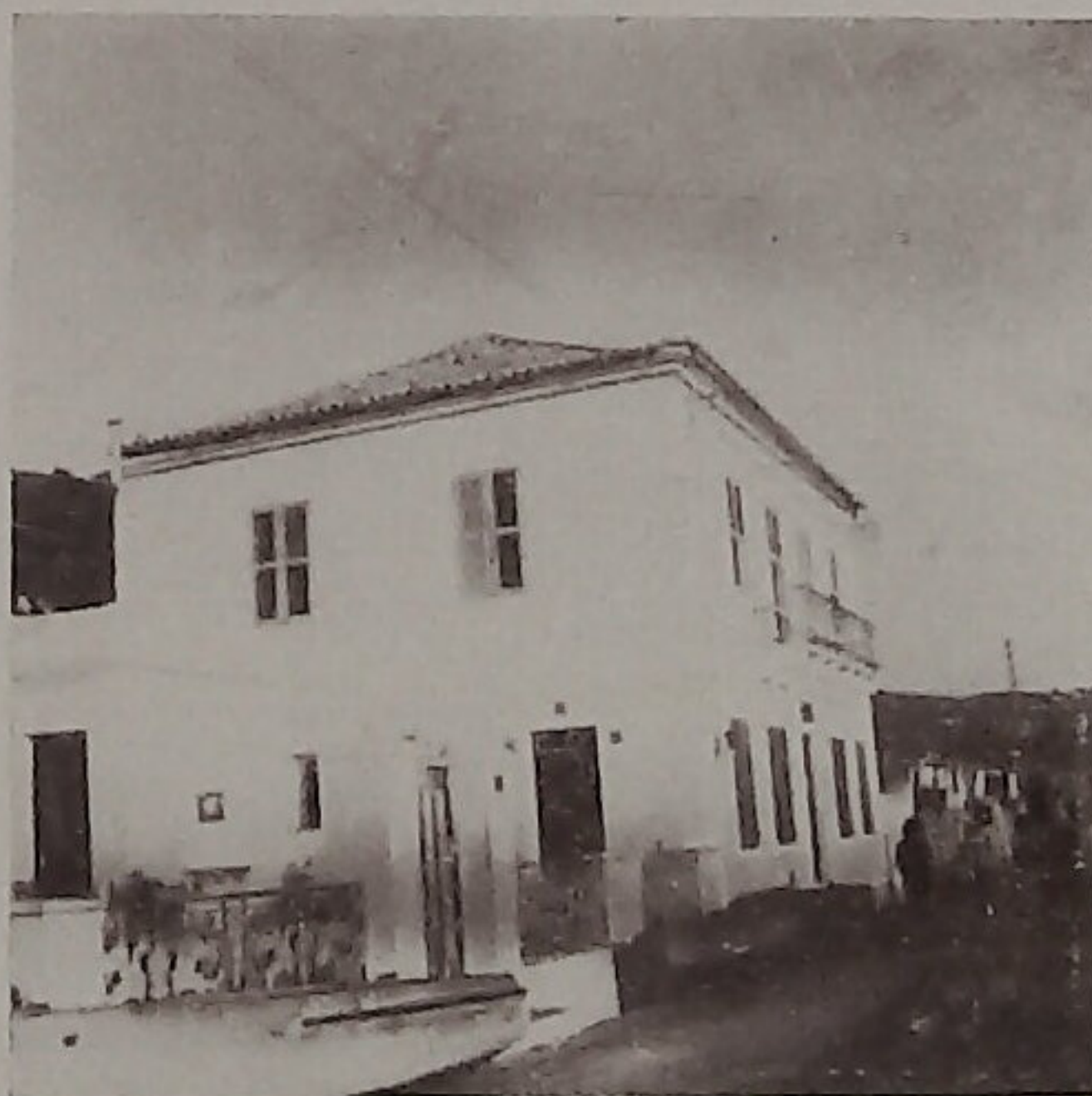
Fig. 15.—One of the three reinforced-concrete buildings in Zante, the municipal school, left intact.
