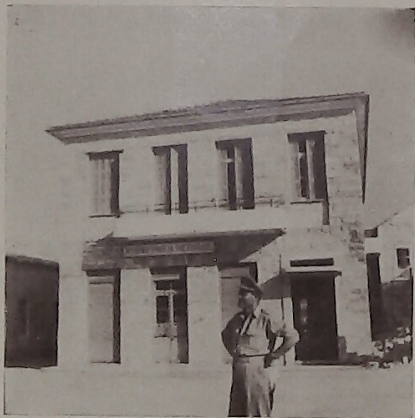
Fig. 14.—A new house of rock construction well built in Vathy (Ithaca), although on made land, left intact.
