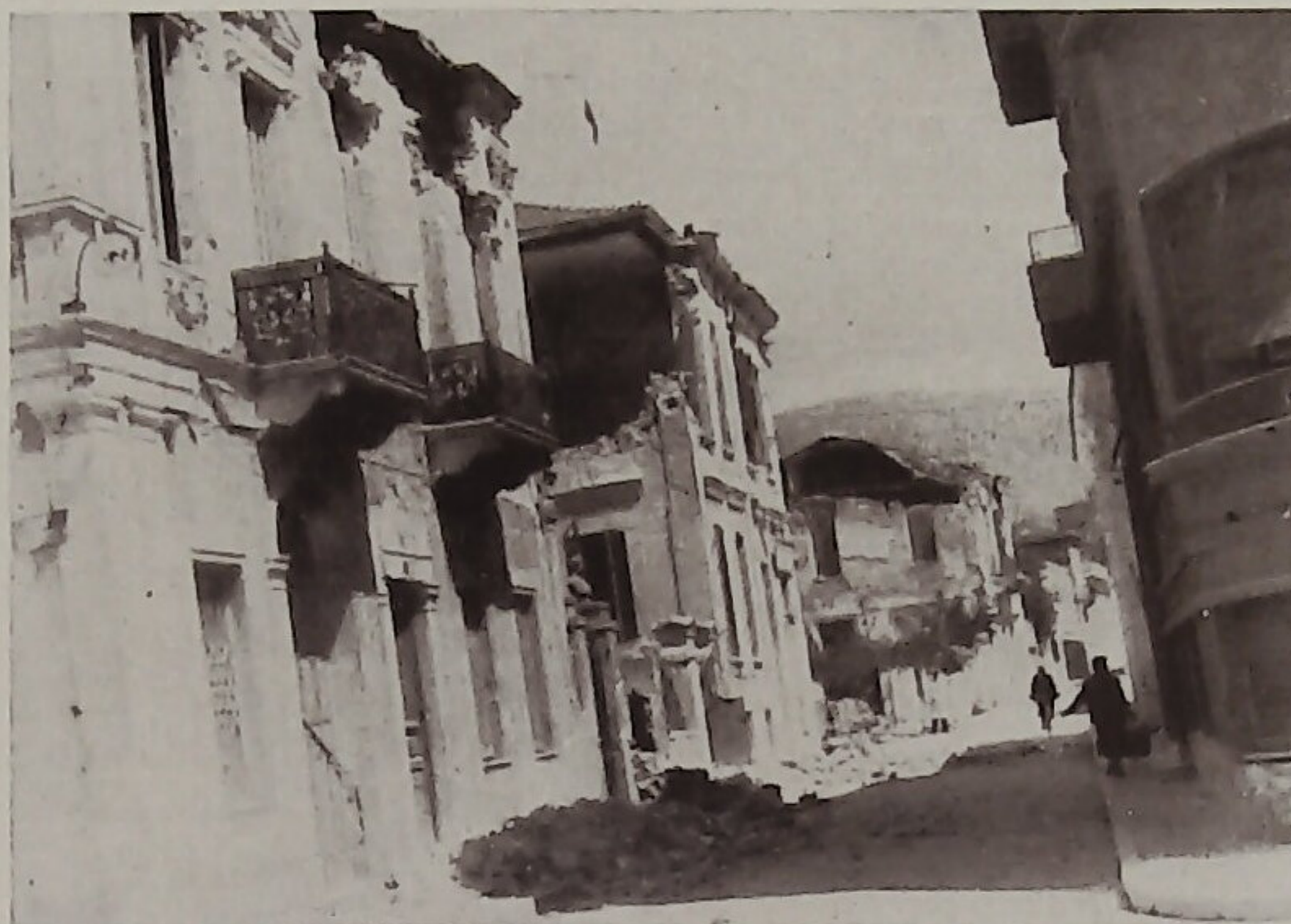
Fig. 1.—A sight of the earthquake failure in Volos after the shocks of April 19 and 21, 1955. Note, that the concrete building on the right hand was left intact.
