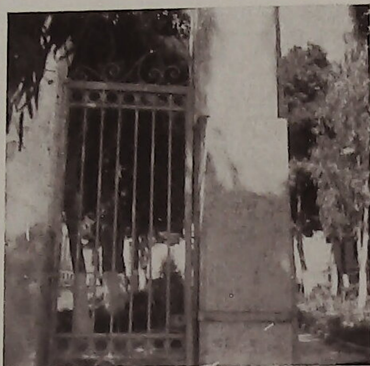
Fig. 7.—The upper part of a column in the entrance of the state hospital, Volos, walked on the lower part during the earthquake of April 19, 1955.
