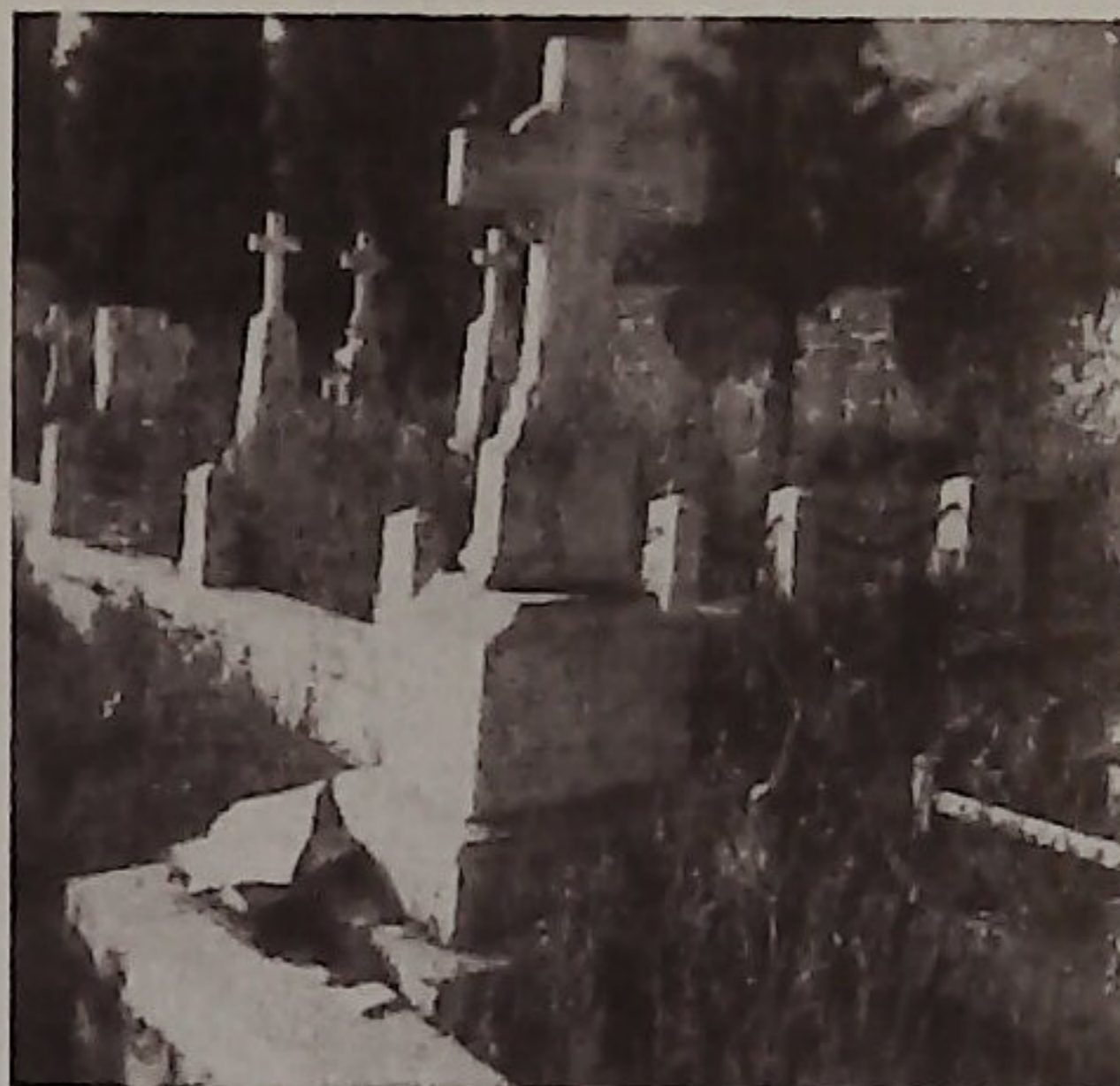
Fig. 16. — Rotation of a tombstone in the cemetery of Agria during the earthquake of April 19, 1955.
