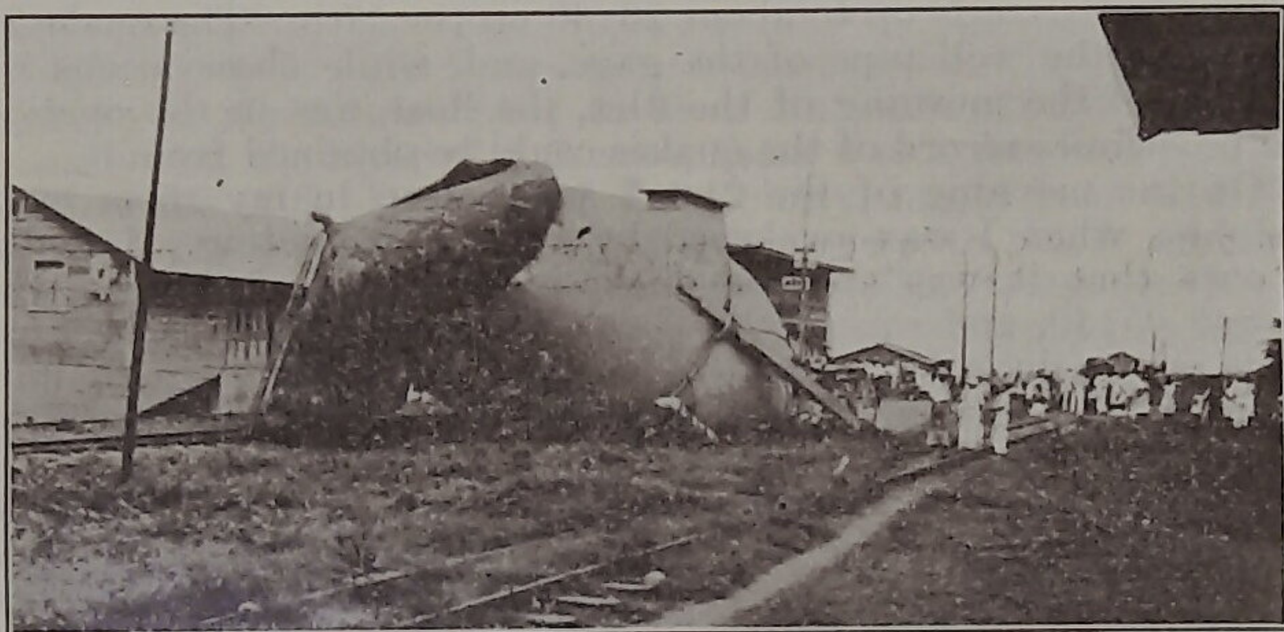
FIGURE 12.—Wrecked water tank. Puerto Armuelles yard. Panama earthquake.
