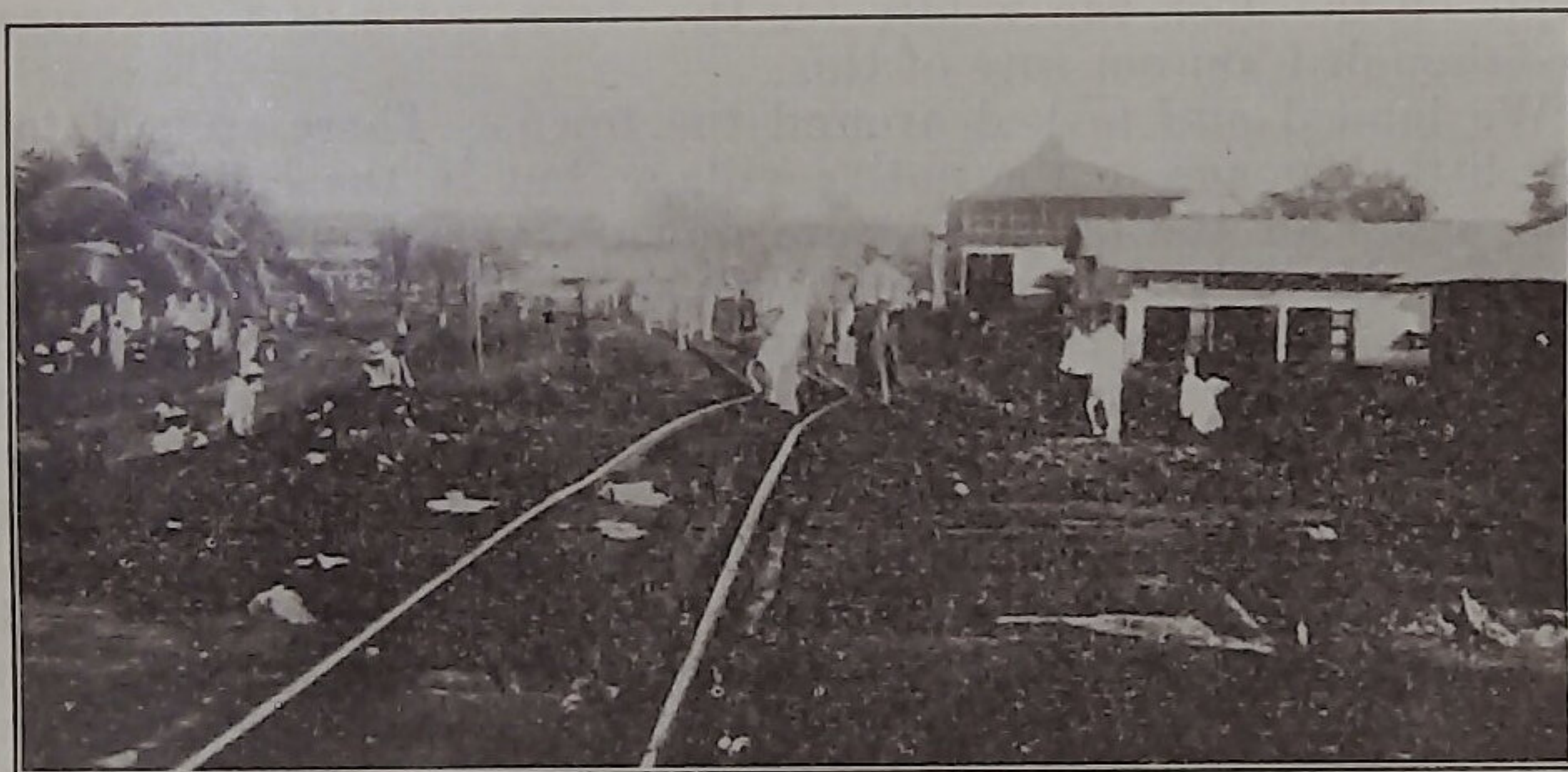
FIGURE 13.—Railroad track shifted out of alinement at Puerto Armuelles. Panama earthquake.
